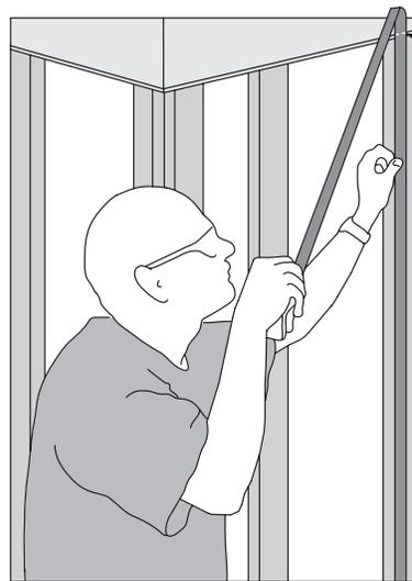
**1** Mark and cut out drywall to fit back and side walls of shower. Remove drywall 1" beyond side wall and top nailing flanges. (Figures 1 and 2)
